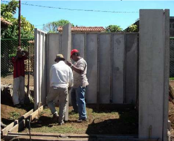
Assembly of ferrocement panels for a core shelter
